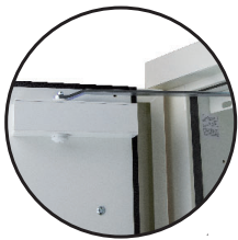
Self-closing door(s) with thermo-fuse
